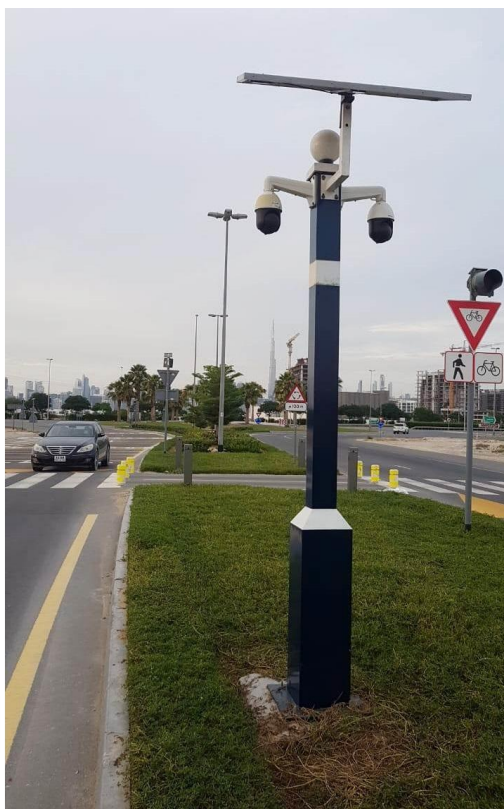
Picture 11: MTP Bicycle Crossing Violation Detector
